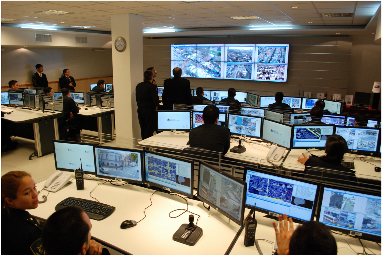
Figure 27: typical video operation room and video operators positions
